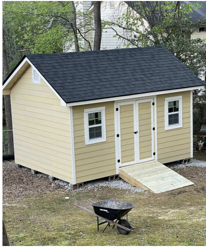
Completed shed with siding, shingles, and ramp access
