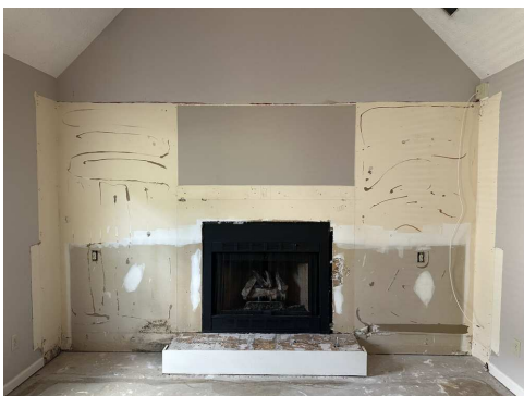
Before — demo down to the original fireplace surround
