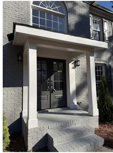
After — finished portico with columns and roofline
