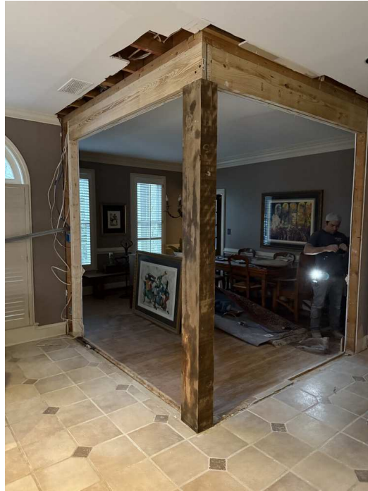
Structural wall removal — framing a header to open a floor plan between rooms
