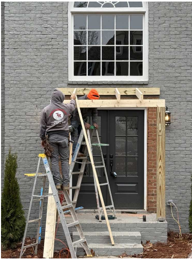
Before — framing the new portico structure
