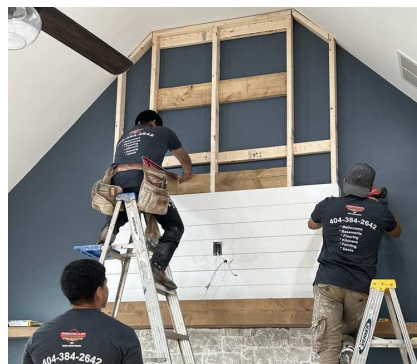
In progress — crew building out the new shiplap feature wall
